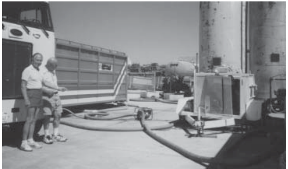
Septic plant on Athens Road in Roseville
